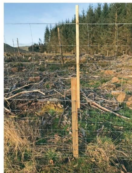
Photo 6. Save costs on deer fencing by using standard livestock fence posts with 1,200mm of rail nailed to them.
